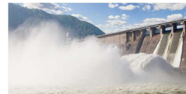
Energy facilities 能源设施
